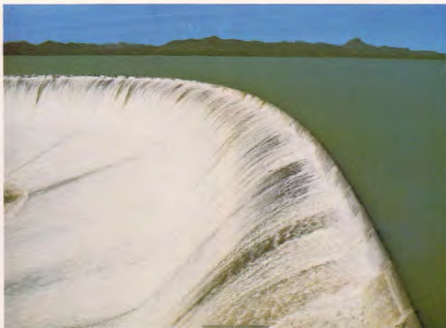
Spillway of the Alvaro Obregón dam (Photo: CIMMYT)
