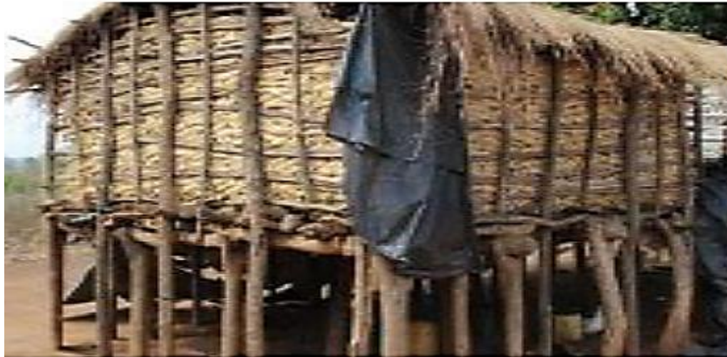
Figure 25. Local granary structure commonly adopted by smallholder farmers for storage of grains in SSA (VIB, 2017).
