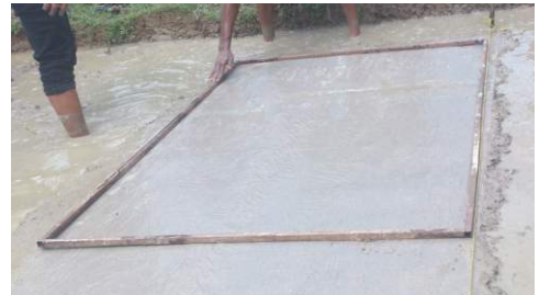
Use an iron frame to help maintain uniform size and thickness of the soil.
