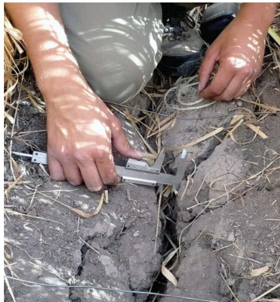
Figure 5. Measurement of crack width.
