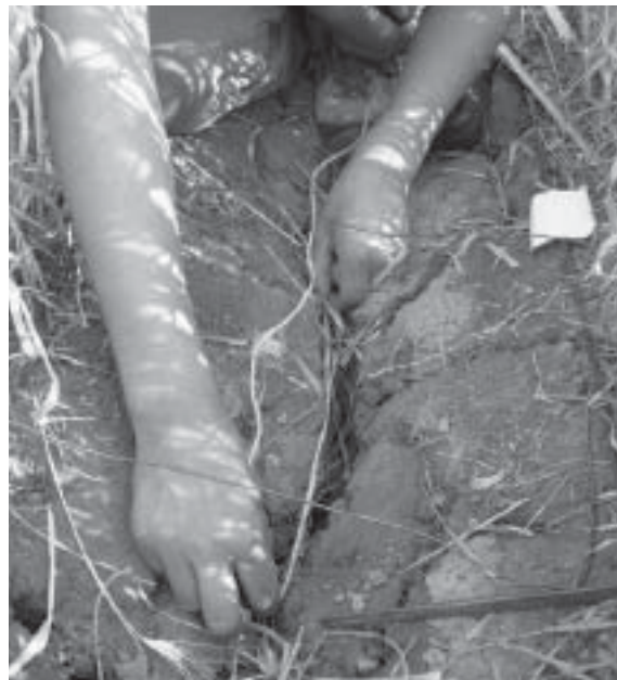
Figure 4. Measurement of crack length.
