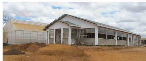
DH facility under development at Kiboko
