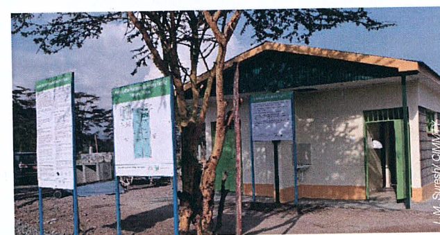
Fig 7: Changing room facility
